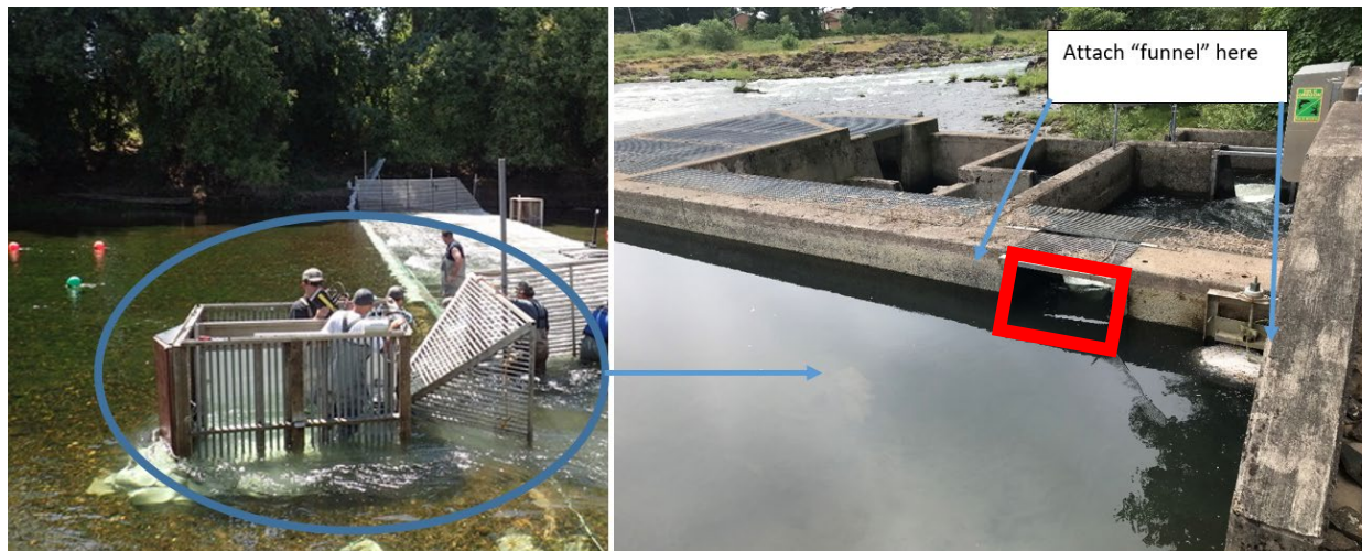
Figure 4 Example of typical VAKI install (Left). "Funnel" and crowder box (circled) could potentially be mounted on the North Bank Ladder(right).
